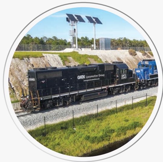
Steel Dynamics supplied premium rail made from recycled scrap for Phase 2 of Brightline's high-speed passenger rail system in Florida.
