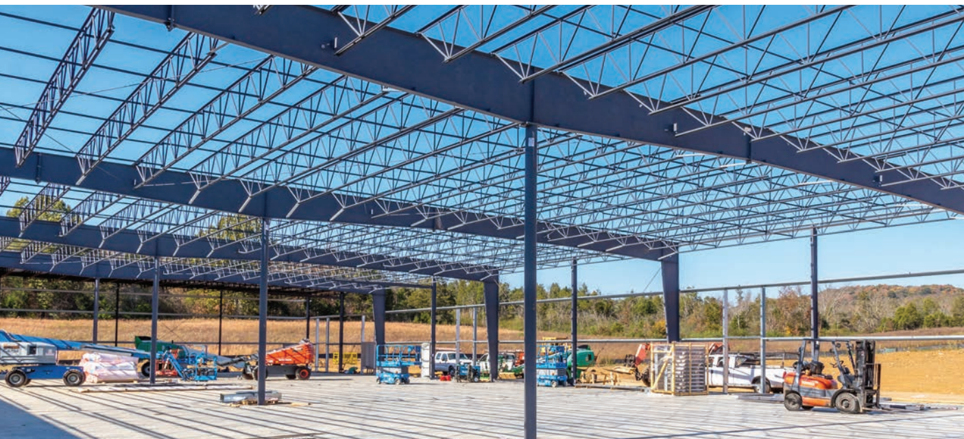
© New Millennium Steel Joist Installation at a Jobsite
